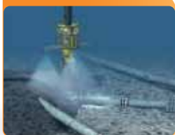
Subsea rock installation
