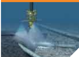
Subsea rock installation
